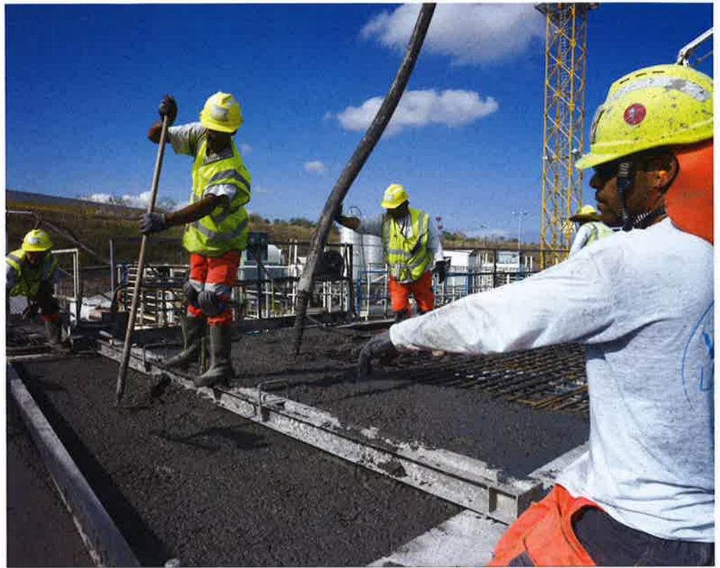
Local labour is employed in the two huge precasting yards
